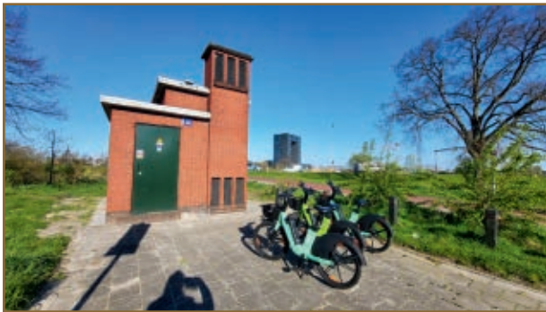
figure 1. The electrical (underground) grid connects several objects in this picture taken in the city of Groningen, The Netherlands: a transformer house from 1936, a modern apartment complex from 2008, and public electric bicycles. In the near future, they will all be part of a CPES through connected DTs in cyberspace.
