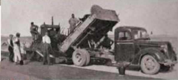
Introduction of machine spreading
