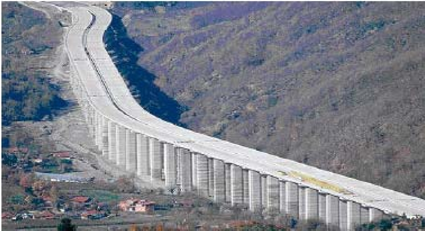
BOLU VIADUCT, TURKEY 2.3 km LONG
