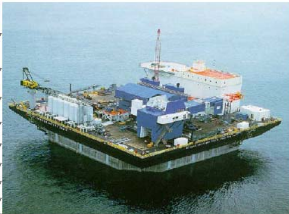
OFFSHORE GAS PLATFORM WITH CONCRETE GRAVITY BASE
