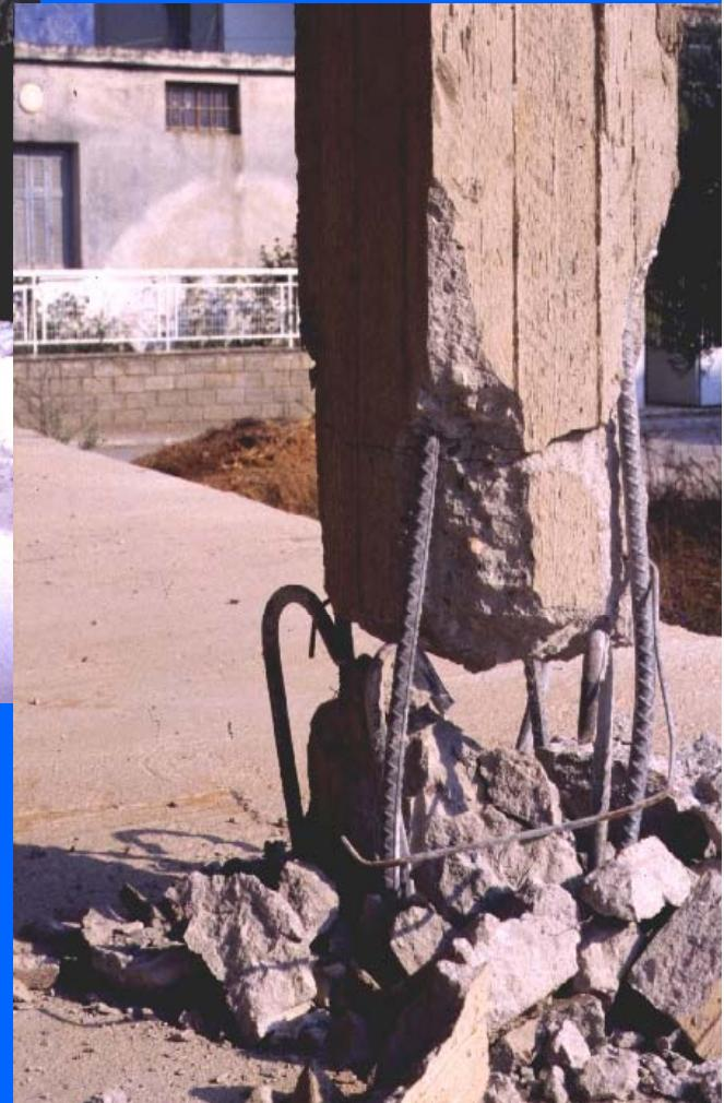
complete disintegration of concrete & buckling of bars in splice zone just above column base
