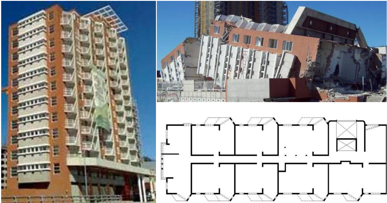
Fig. 2.13 Collapse of Alto Rio wall building in Concepción, Chile; February 2010 earthquake (structural walls are shown in black in the framing plan).
