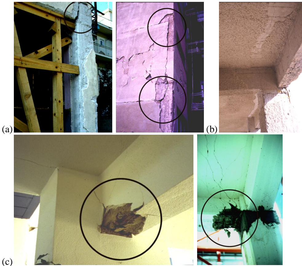
Fig. 2.22 Typical features of beam behaviour: (a) pullout of beam bars from narrow corner column, due to short straight anchorage there; (b) wide crack in slab at right angles to the beam at the connection with the columns shows the large participation of the slab as effective flange width in tension; (c) failure, with concrete crushing and bar buckling at bottom flange next to the column.
