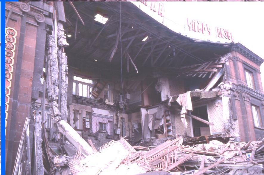
Collapse of buildings w/ precast concrete floors inadequately connected to the walls (Armenia, 1988)
