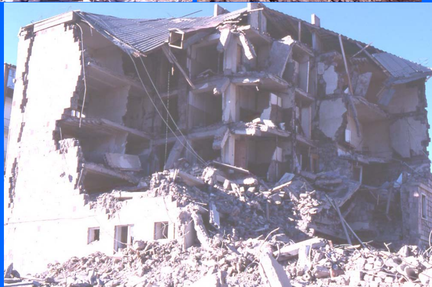
Collapse of buildings w/ precast concrete floors inadequately connected to the walls (Armenia, 1988)
