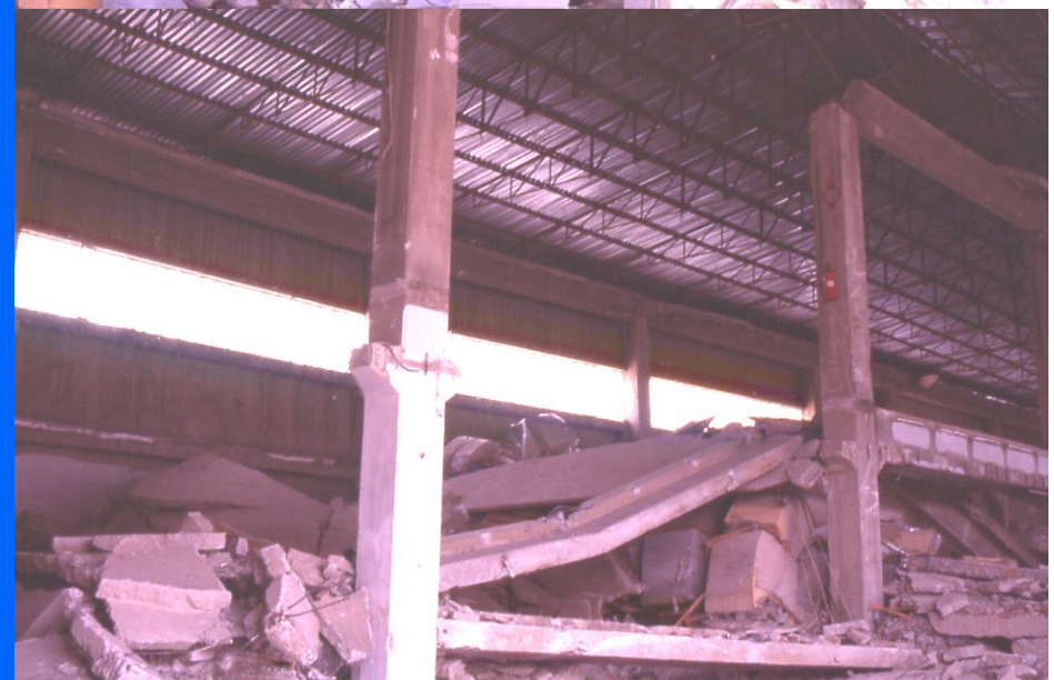
Collapse of precast building, w/ floors poorly connected to lateral-load-resisting system (Athens, 1999).
