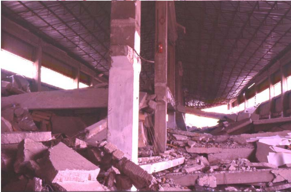
Collapse of precast building, w/ floors poorly connected to lateral-load-resisting system (Athens, 1999).
