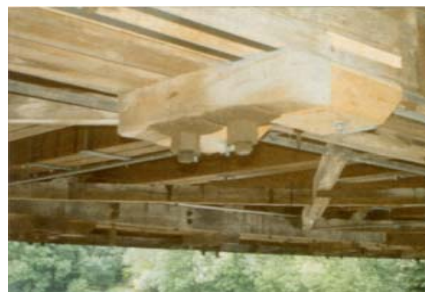
Murgenthal-Fulenbach Timber Bridge (1864)
