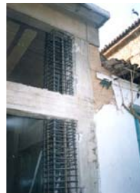
ADDITION OF SHEAR WALLS
