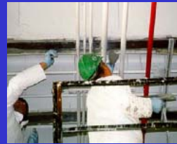
Removal of excess resin
