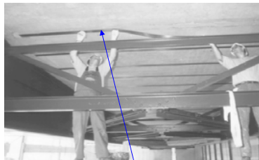
Slab flexural strengthening
