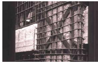
STEEL PLATES & SHOTCRETE JACKETING
