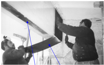
Beam flexural strengthening with strips
