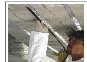
FRP inside slits (NSM)
