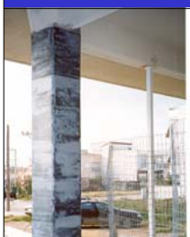
Column wrapping with fabrics
