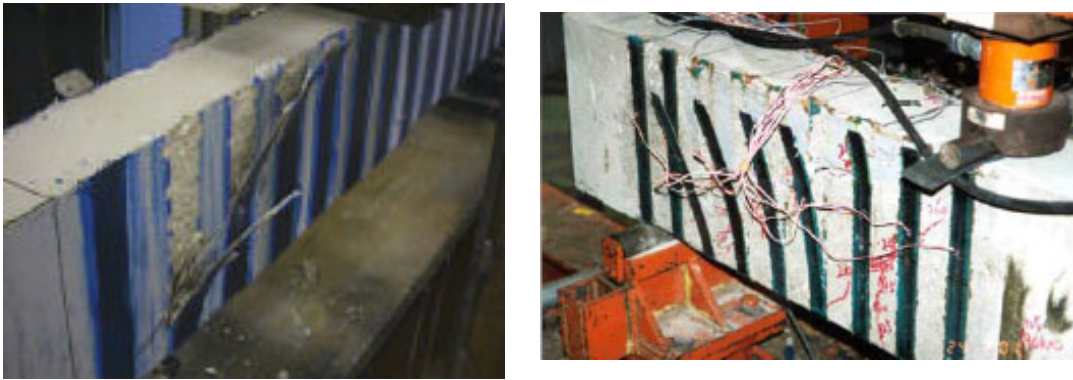
Fig. 5.5 Debonding of FRP strips used for shear strengthening.
