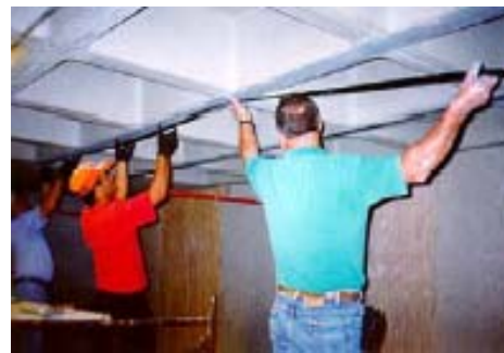
Placement of strip.
