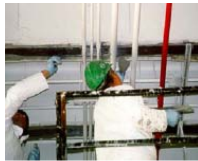
Removal of excess resin.
