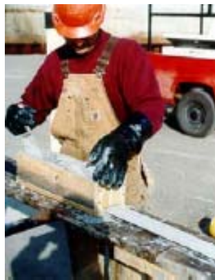
Resin application on strip.
