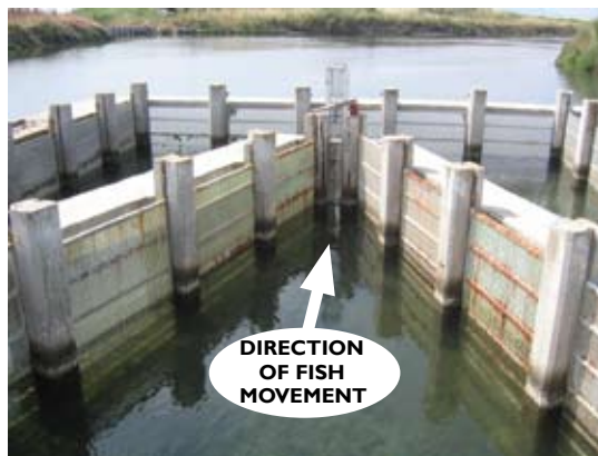
Figure 2: Permanent fish entrapment devices, which catch live fish as they move seawards (Vassova and Erateino Lagoons, Nestos Delta). The arrow shows the direction of fish movement. Source: E.T. Koutrakis.
