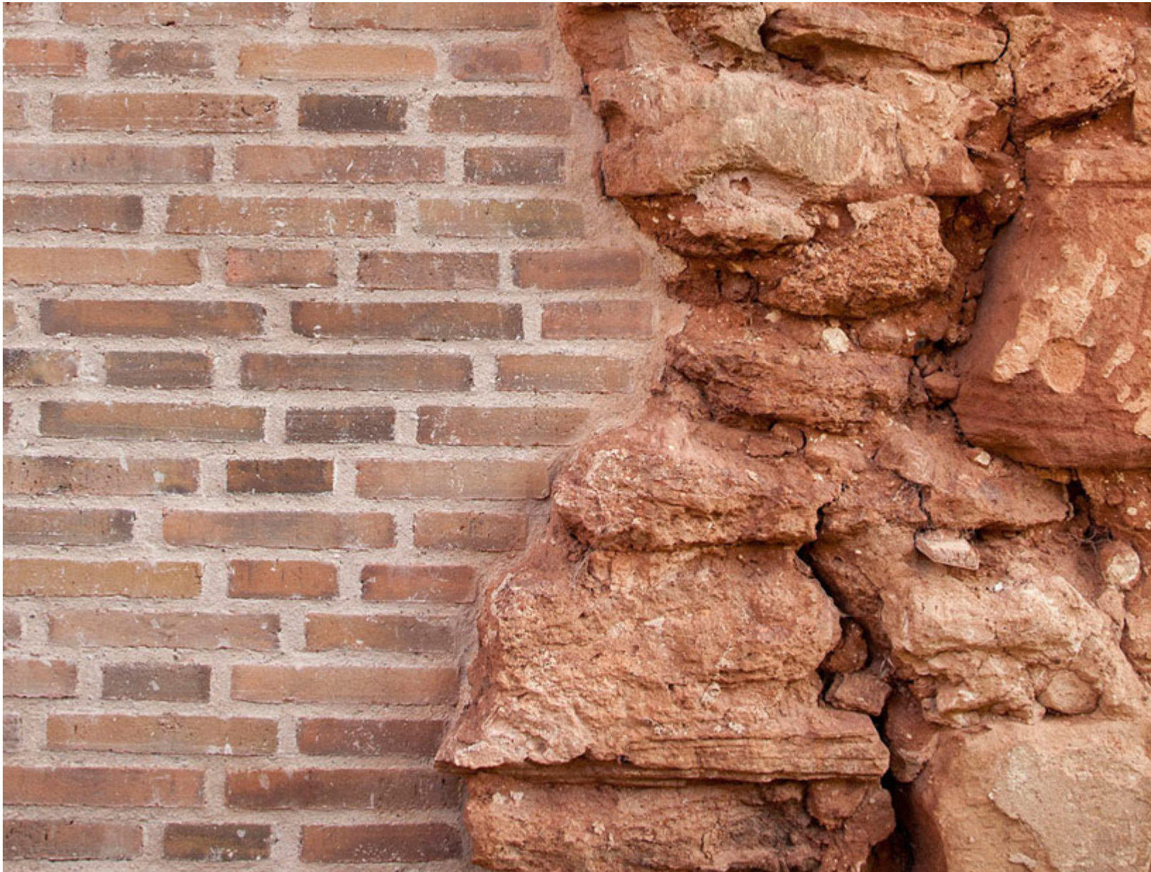
bricks follow the uneven wall lines of the original masonry walls
