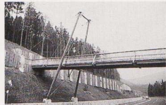
Diagonal cable construction with raking pylon
