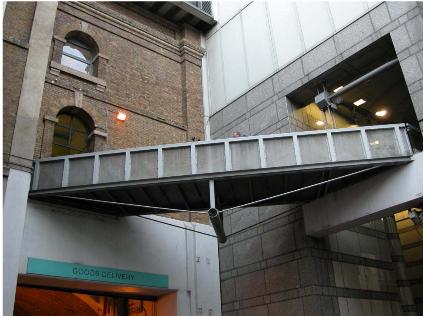
with two posts and beam in bending under asymmetric loading
