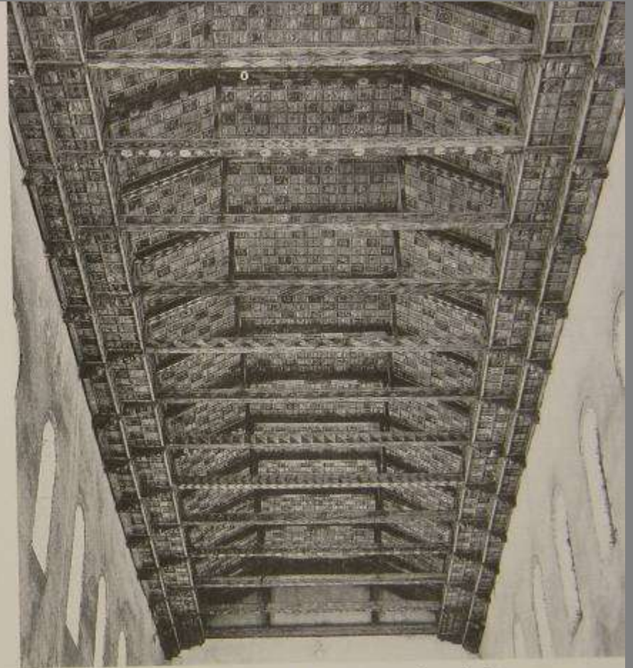
Roof truss of the San Francesco church, Ravenna
