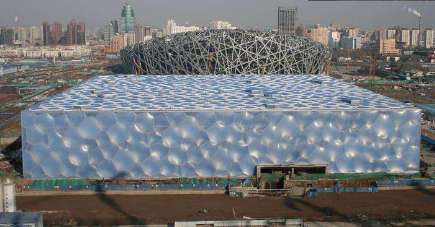
Beijing National Aquatics Centre, PTW Architects, 2008
