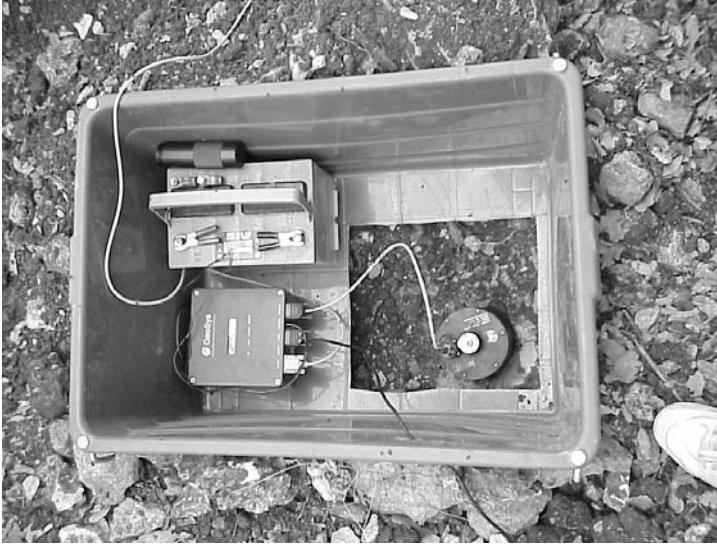
Figure 7.12 A very simple field installation. A plastic box has been placed directly on the ground. The sensor is placed in the cut out hole. Inside are also the battery and recorder. The cable going out is for the GPS. After installation, soil was put up around the sides and insulation was put on top of the lid. The sensor is a Kinemetrics Ranger 1 Hz seismometer (Table 2.3) and the recorder is a GeoSIG GBV316 (Table 5.3).
