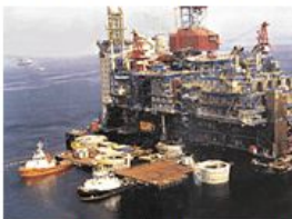
Sinking of Sleipner A offshore platform, 1991 (700M because of inaccurate fem approximation)
