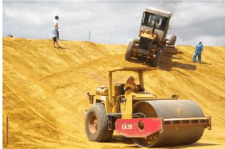
Compaction of the slopes with the help of a compactor
