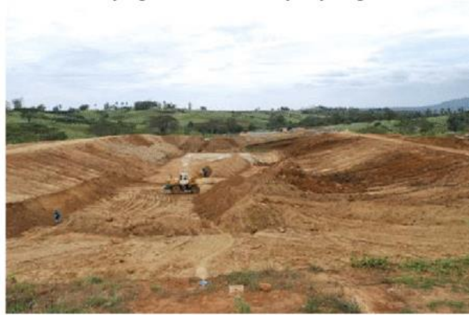
Surveying of the first cell by city engineers
