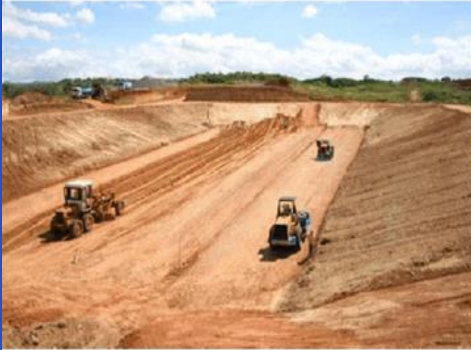
Compaction of the clay liner
