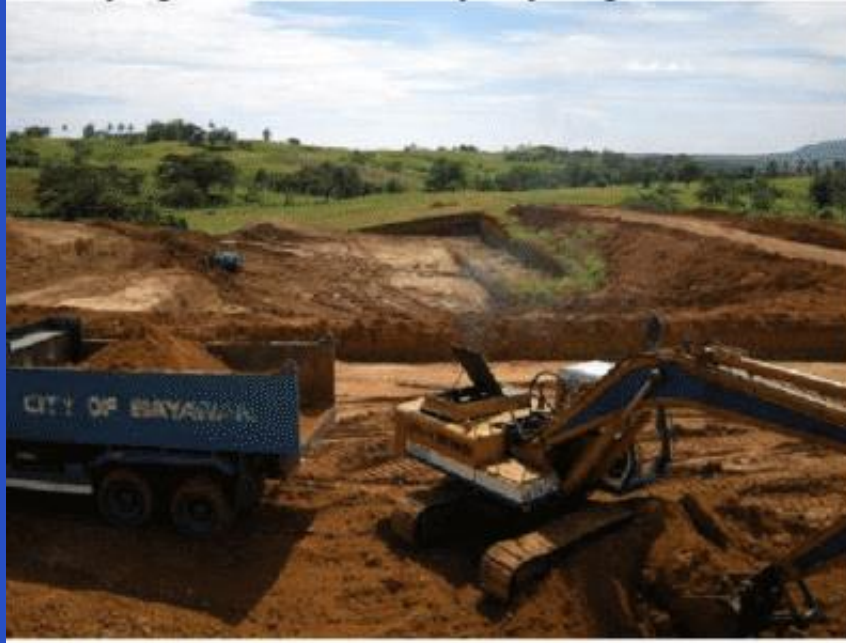
Surveying of the first cell by city engineers
