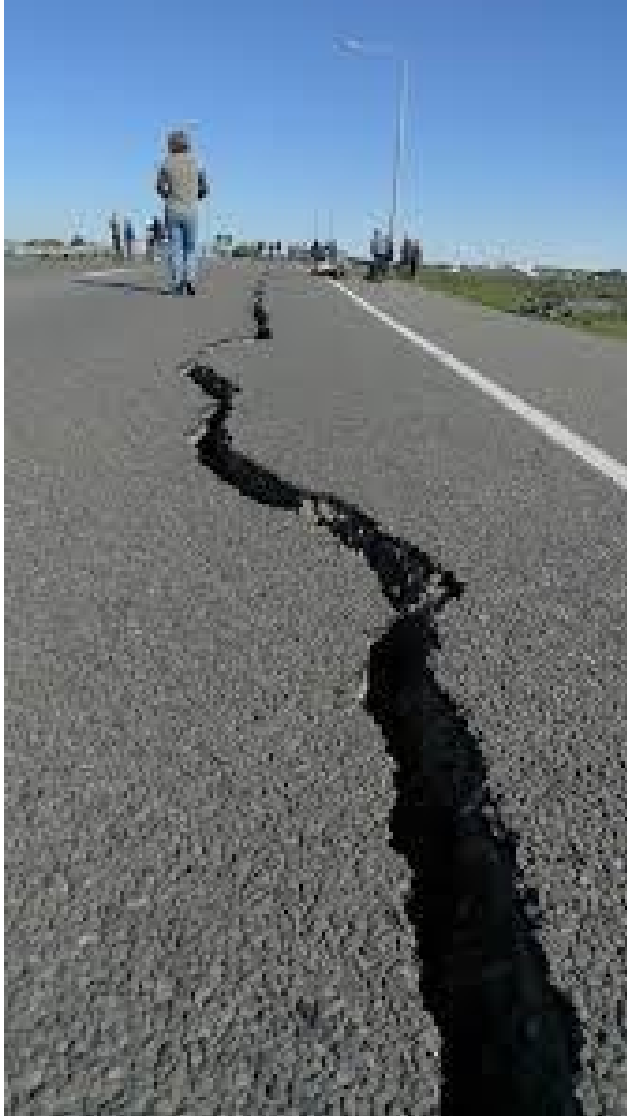
http://en.wikipedia.org/wiki/2010_Canterbury_earthquake#/media/File:Crack_in_Bridge_Street_from_the_2010_Canterbury_earthquake.jpg Crack in Bridge Street, South New Brighton.
