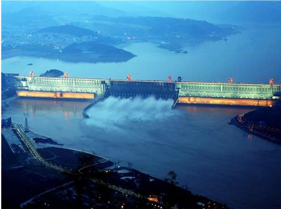
Three Gorges Dam (China)
