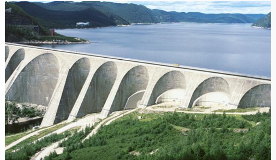
Daniel-Johnson Dam (Canada)
