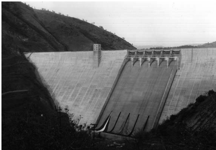
Figure 2.1.2d Pine Flat Dam on the Kings River, near Fresno, California. The fundamental natural vibration period of this 122-m-high concrete gravity dam was measured by forced vibration tests to be 0.288 s and 0.306 s with the reservoir depth at 94.5 m and 105 m, respectively.
