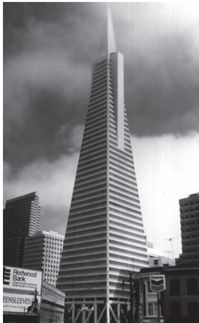
Figure 2.1.2b Transamerica Building, San Francisco, California. The fundamental natural vibration periods of this 49-story steel building, tapered in elevation, are 2.90 s for north–south vibration and also for east–west vibration. These vibration properties were determined by forced vibration tests. (Courtesy of International Structural Slides.)
