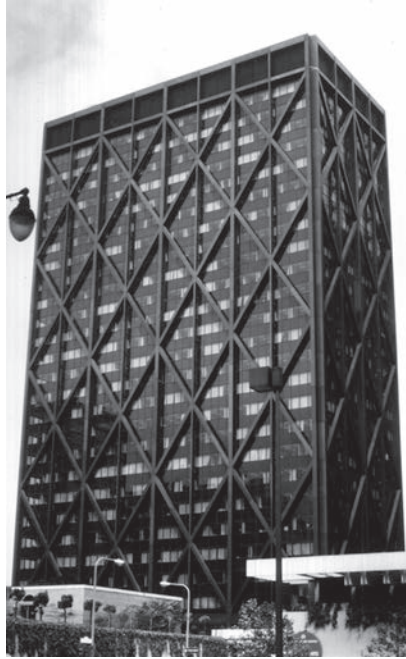
Figure 2.1.2a Alcoa Building, San Francisco, California. The fundamental natural vibration periods of this 26-story steel building are 1.67 s for north–south (longitudinal) vibration, 2.21 s for east–west (transverse) vibration, and 1.12 s for torsional vibration about a vertical axis. These vibration properties were determined by forced vibration tests. (Courtesy of International Structural Slides.)
