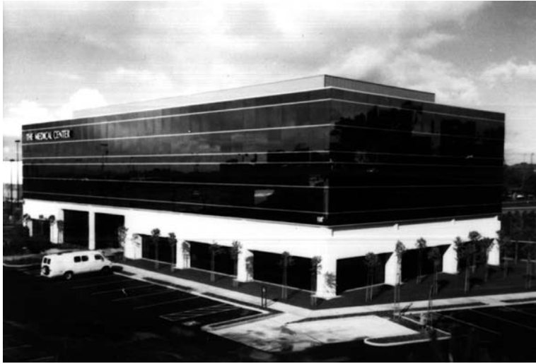
Figure 2.1.2c Medical Center Building, Richmond, California. The fundamental natural vibration periods of this three-story steel frame building are 0.63 s for vibration in the long direction, 0.74 s in the short direction, and 0.46 s for torsional vibration about a vertical axis. These vibration properties were determined from motions of the building recorded during the 1989 Loma Prieta earthquake. (Courtesy of California Strong Motion Instrumentation Program.)
