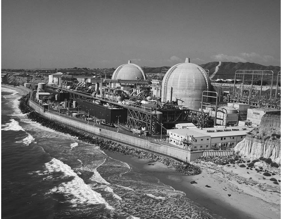
Figure 1.10.1 These two reinforced-concrete dome-shaped containment structures house the nuclear reactors of the San Onofre power plant in California. For design purposes, their fundamental natural vibration period was computed to be 0.15 s assuming the base as fixed, and 0.50 s considering soil flexibility. This large difference in the period indicates the important effect of soil–structure interaction for these structures. (Courtesy of Southern California Edison.)
