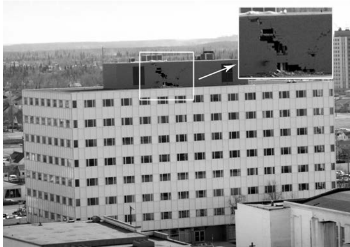
Figure 13.2.12 The Hill Building in Anchorage, Alaska, after the Prince William Sound earthquake, March 27, 1964, Magnitude 9.2. Except for the damage to the penthouse wall (close-up), the building was essentially undamaged. (From the Steinbrugge Collection, National Information Service for Earthquake Engineering, University of California, Berkeley.)
