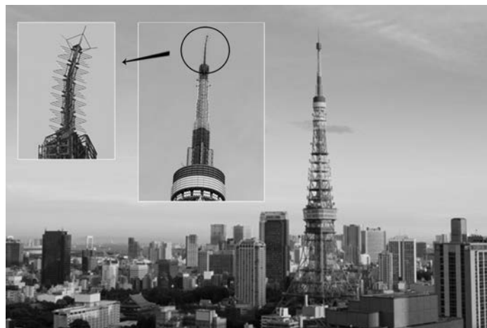
Figure 13.2.13 The 332.5 m-high Tokyo Tower performed well during the Tohoku, Japan, earthquake, March 11, 2011, Magnitude 9.0, except that the top part bent permanently. Shown is the tower before and after, with a second focus on the bend near the top. (Courtesy of C. D. James and C. Bodnar-Anderson, National Information Service for Earthquake Engineering, University of California, Berkeley.)
