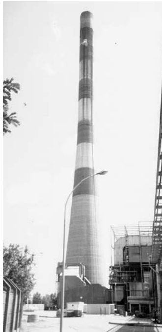
Figure 2.1.2f Reinforced-concrete chimney, located in Aramon, France. The fundamental natural vibration period of this 250-m-high chimney is 3.57 s; it was determined from records of wind-induced vibration.
