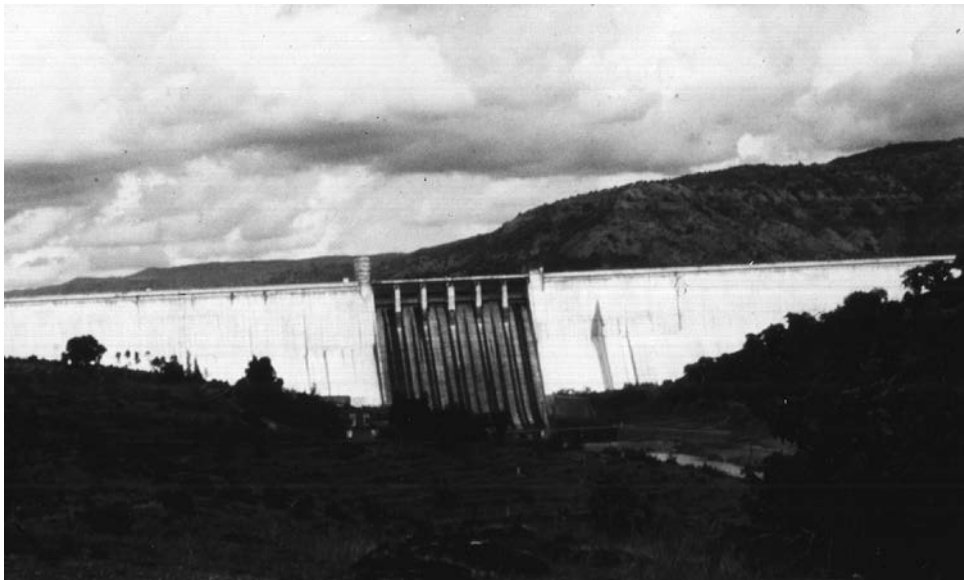
Figure 18.11.3 Koyna Dam, a 103-m-high and 853-m-long concrete gravity dam near Poona, India. This major dam was damaged by the Koyna earthquake of December 11, 1967, a Magnitude 6.5 event centered 4.8 km from the dam. [From A. K. Chopra, "Earthquake Response Analysis of Concrete Dams," in Advanced Dam Engineering for Design, Construction and Rehabilitation (ed. R. B. Jansen), Van Nostrand Reinhold, New York, 1988.]
