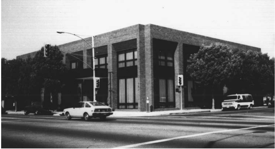
Figure 13.4.1 First Federal Savings building, a two-story reinforced-concrete building (with a partial basement) in Pomona, California. (Courtesy of California Strong Motion Instrumentation Program.)
