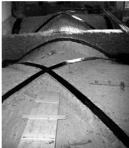
Fig. 2.6 Examples for the application of the basic FRP strengthening technique.
