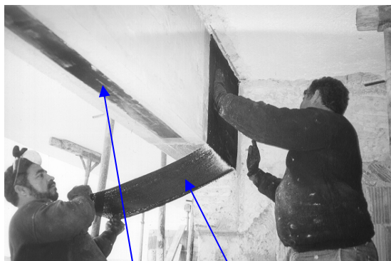
Hand lay-up of CFRP strip
