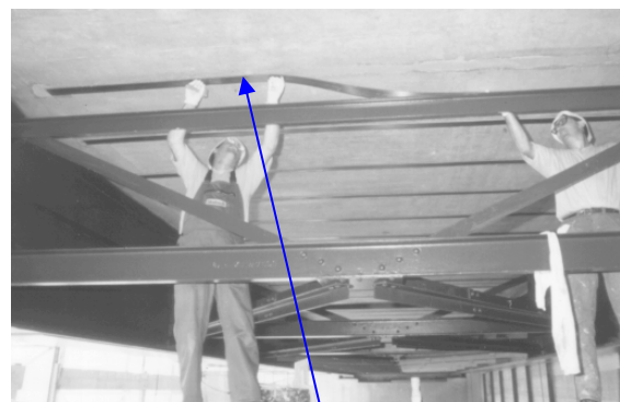
Flexural strengthening of bridge deck using CFRP strips
