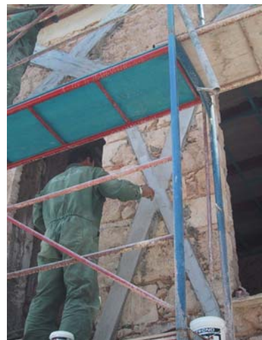
Preparation (levelling) of masonry substrates for the bonding of CFRP strips
