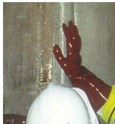
Application of pre-impregnated fabric
