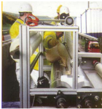
Impregnation of fabric with epoxy resin
