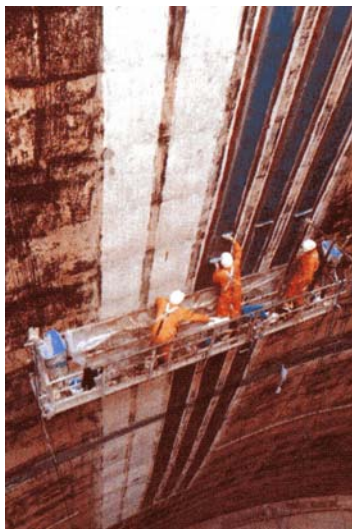
Strengthening of cooling tower with carbon fabrics
