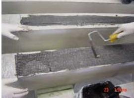
Epoxy-bonded textile (FRP)
