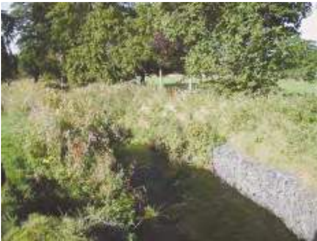
E1Ka Gabion bank material – boulders/cobbles in wire baskets. Typical example of use in protection of the bottom half of a bank.
