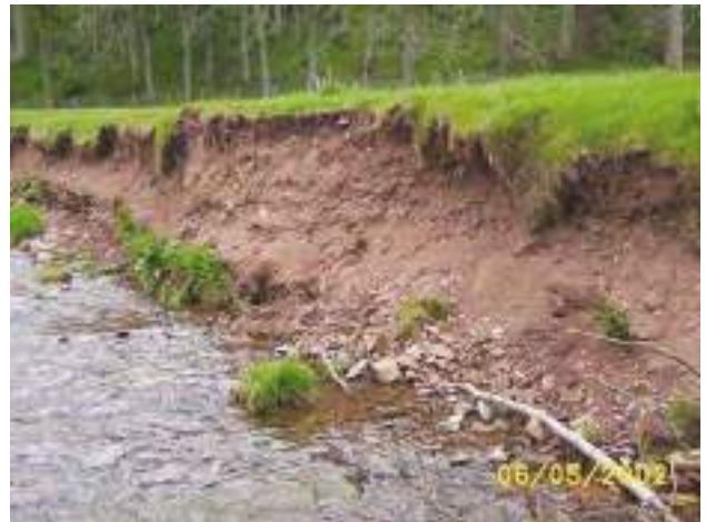
E1Eb Earth bank material; a 'jab' with the ranging pole will not leave a smooth, well-defined, hole.
