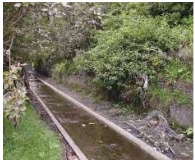
E4Jb Artificial channel substrate – concrete bed.
