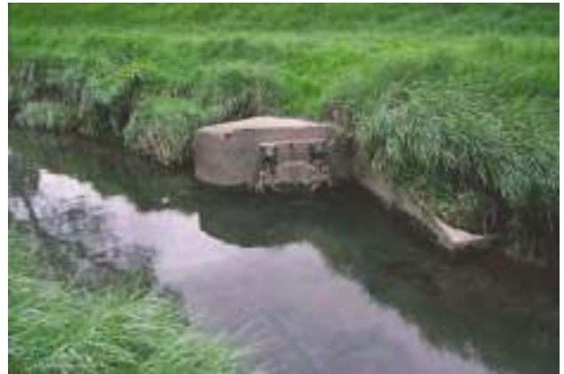
D4c Minor outfall – example of a flap-valve on a drainage channel – all such structures occupying <10m bank-length are recorded as ‘minor’.
