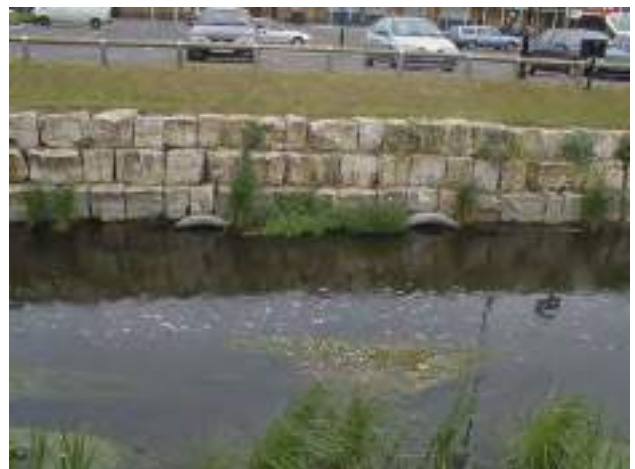
E1Mb Rip-rap bank material; placed (but not cemented), square, blocks. Note under-water 'pipes' for fish shelter (note in Section P).
