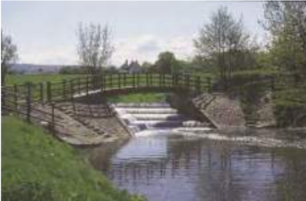
D1a Major weir/sluice – weir; has a fixed level. This is an example of a composite weir. Note also to record a minor bridge. Flow-type is ‘chute’. It is essential to photograph all major structures to aid interpretation of probable impact.
