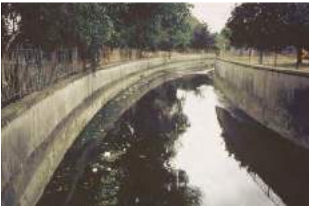
E1Ha Concrete bank material. See also A1c, E2Cb, E7Cc.
