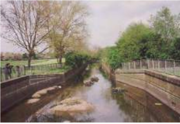
E7Cc Unvegetated mid-channel bar – example in urban stream. Note concrete bank material and presence of shopping trolleys (urban debris; but not predominant).
