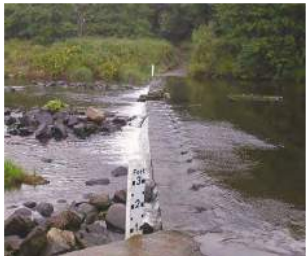
D5a Major ford – both the bed and banks are made of artificial material, and there is obvious ponding of water upstream.
