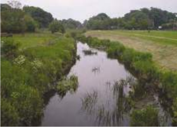
E2Aa Resectioned (reprofiled) bank – tell-tale smooth (trapezoidal) slope even though undertaken many years ago; river also over-deepened, with tell-tale ‘step’ in the profile where bed material at the base of the bank removed. See also A1a, D8a,b,c, E3Da, I6b.
