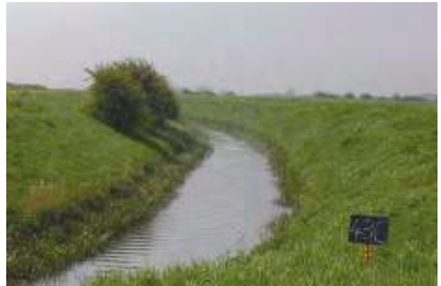
E6e Resectioned bank – this example shows river with few trees, very even gradients to the banks, and with the banktop width <math>< 4</math> times the banktop height indicating both deepening and resectioning.
