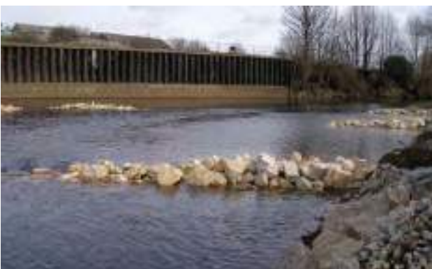
D6e Minor deflector/groyne/croy – extends across <10% of the channel width. Example of boulder deflector installed to improve fish habitat.
