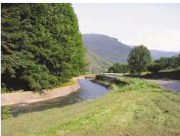
A1c Concrete channel replacing part of natural watercourse; site is obviously hugely modified but is still part of a river. Note road on right hand side (suburban land-use).
