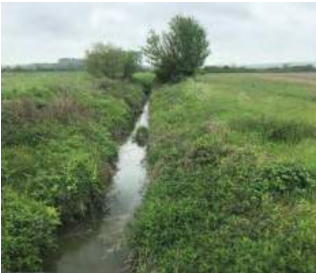
D7b An obviously realigned channel.
