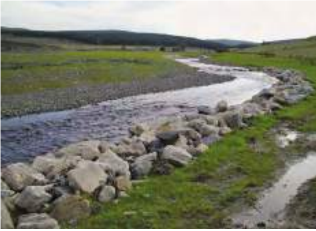
E1Mc Rip-rap bank material; tipped boulders.
