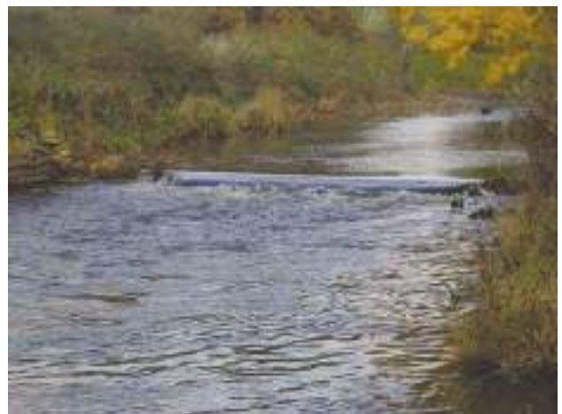
D9a Is water impounded by weir/dam? Photo shows water artificially impounded behind a shallow weir structure. See also D1b,c, D5a.
