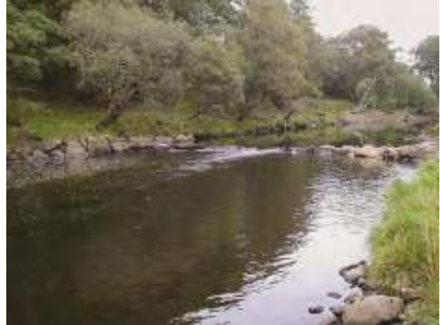
D1e Intermediate weir – boulders are not cemented, and water can leak through the fissures.
