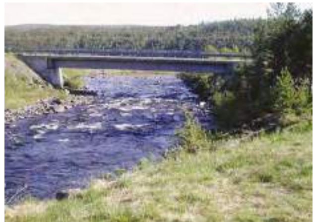
D3c Intermediate bridge – no central piers, and with bank-side abutments 10-25m long. Note broken standing waves.
