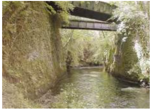
D3b Major bridge – all bridges with bankside abutments >25m long.
