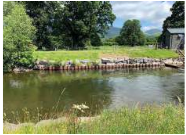
16b Reinforced bank – toe only; reinforcement is metal sheet piling and rip rap above. Note also bank is resectioned.
