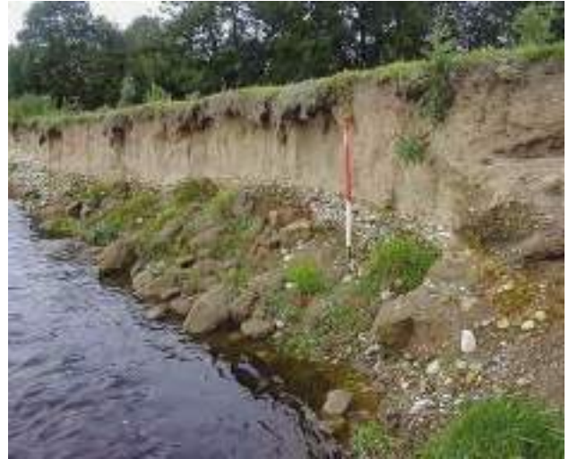
I2b Vertical plus toe bank profile. Note bank is eroding cliff with sandy/gravel soil (EC).
