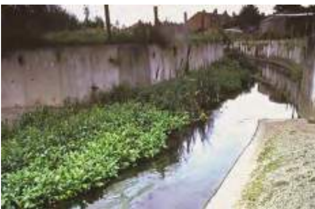
E1Hb Concrete bank material. This example illustrates an artificial berm as habitat creation as part of a flood defence scheme, and this should be noted in Section P.
