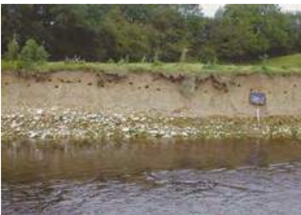
E1Dc Gravel/sand bank material – example with mixed materials, but gravel/sand predominates. Note in Section P use of bank by sand martins.
