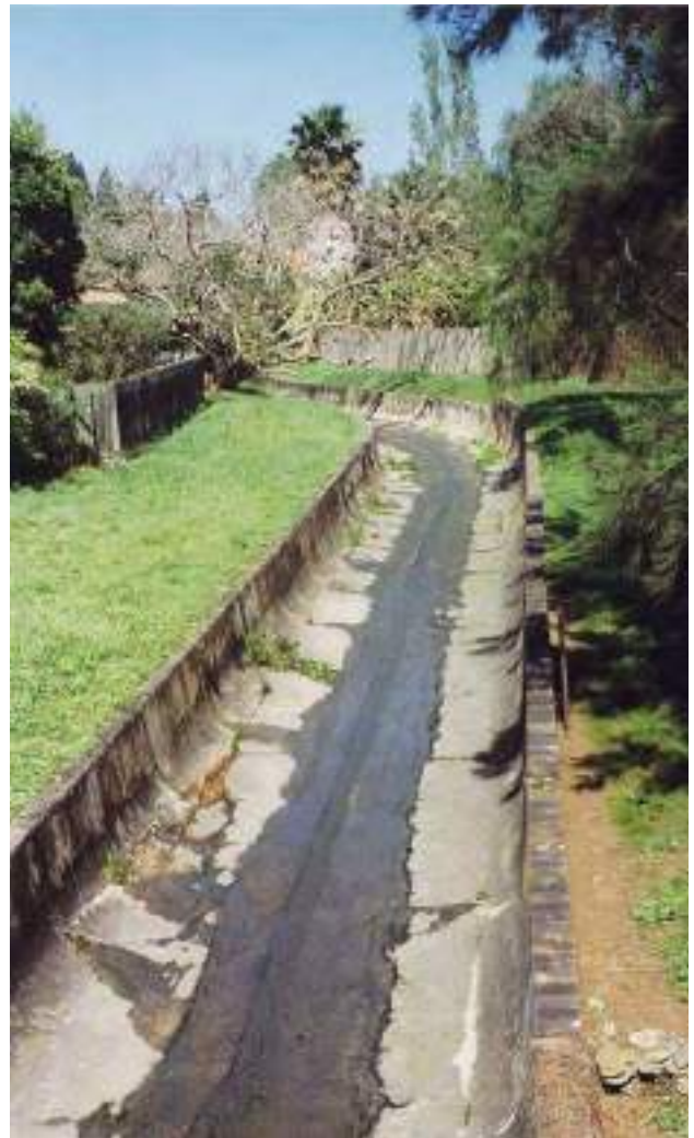
E4Ja Artificial channel substrate – both bed and banks artificial. See also D5a,b, E1La.
