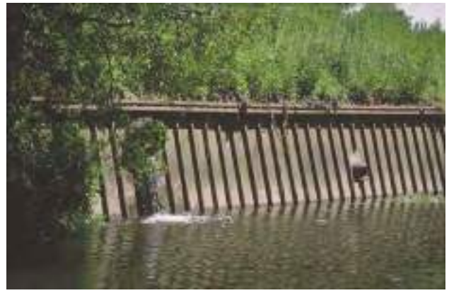
E1Ia Sheet piling bank material.
