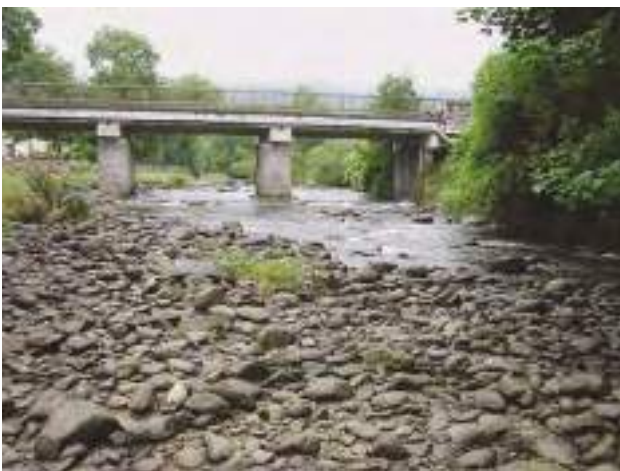
D3a Major bridge – all bridges with central piers are classed as ‘major’. Note importance of photographs to show size of piers, and degree of associated bed armouring. Classic cobble channel substrate exposed in foreground. See also D5b.
