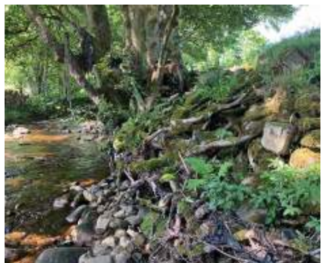
J9b Exposed bankside tree roots.
