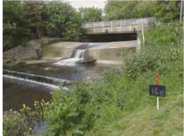
D1d Major weir/sluice – example of a complex weir structure used for measuring flow. Note also an intermediate bridge.
