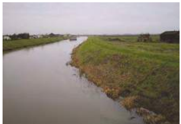
E2Da Embanked – note the earth embankment is placed on top of the natural bank (cf. set-back embankment, Section I).
