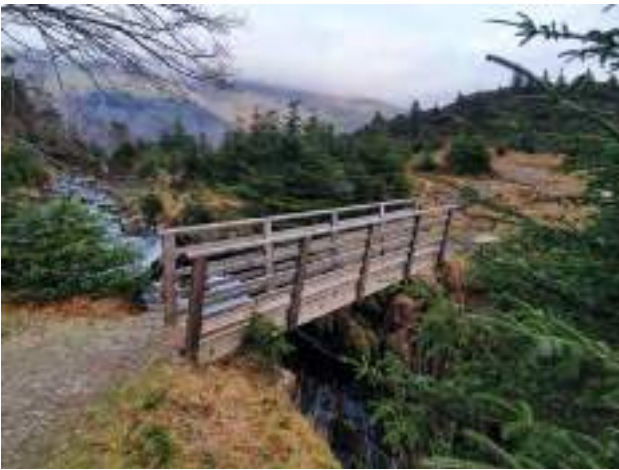
D3f Minor bridge – bridge lacks in-channel supports and has bank abutments <10m wide.
