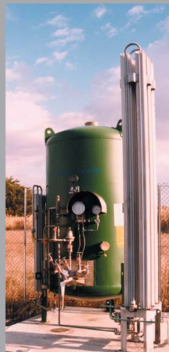
Fig.58.01 Small liquid oxygen reservoir sized for hatchery need (photo STM Aquatrade)
