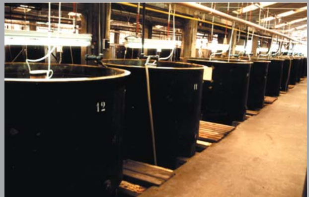
Fig.43.02 An outdated hatchery layout were eggs incubates directly in the tanks (photo M. Caggiano)
