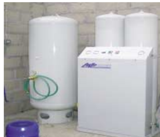
8 Oxygenation In intensive production systems, the rate of oxygen consumption by fish and bacteria may exceed the capabilities of typical aeration equipment. In order to maintain a high carrying capacity, pure gaseous oxygen injection is used to allow a higher availability of Oxygen
