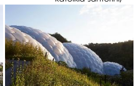
Eden project biomes, Grimshaw and Partners, 2001, Cornwall https://grimshaw.global/projects/the-eden-project-the-biomes/
