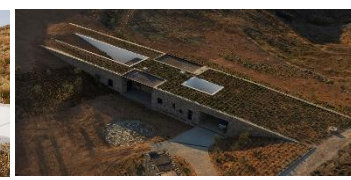
Aloni | DECA architecture | 2008 Avriparos https://deca.gr/project/aloni/
