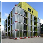
Bioadaptive façade BIQ Αμβούργο Γερμανία https://99percentinvisible.org/article/architectural-ecosystems-bioreactors-generate-green-energy-shade-oxygen/
