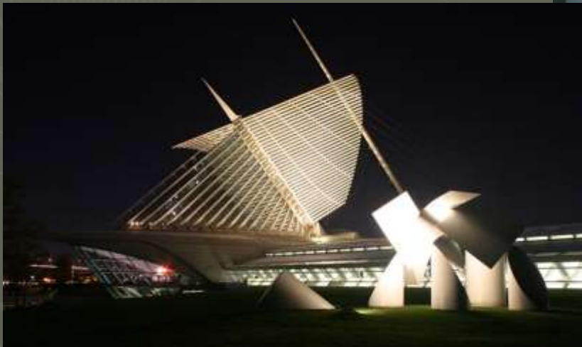
Milwaukee Art Museum, Wisconsin, U.S.A., Santiago Calatrava, 2001
