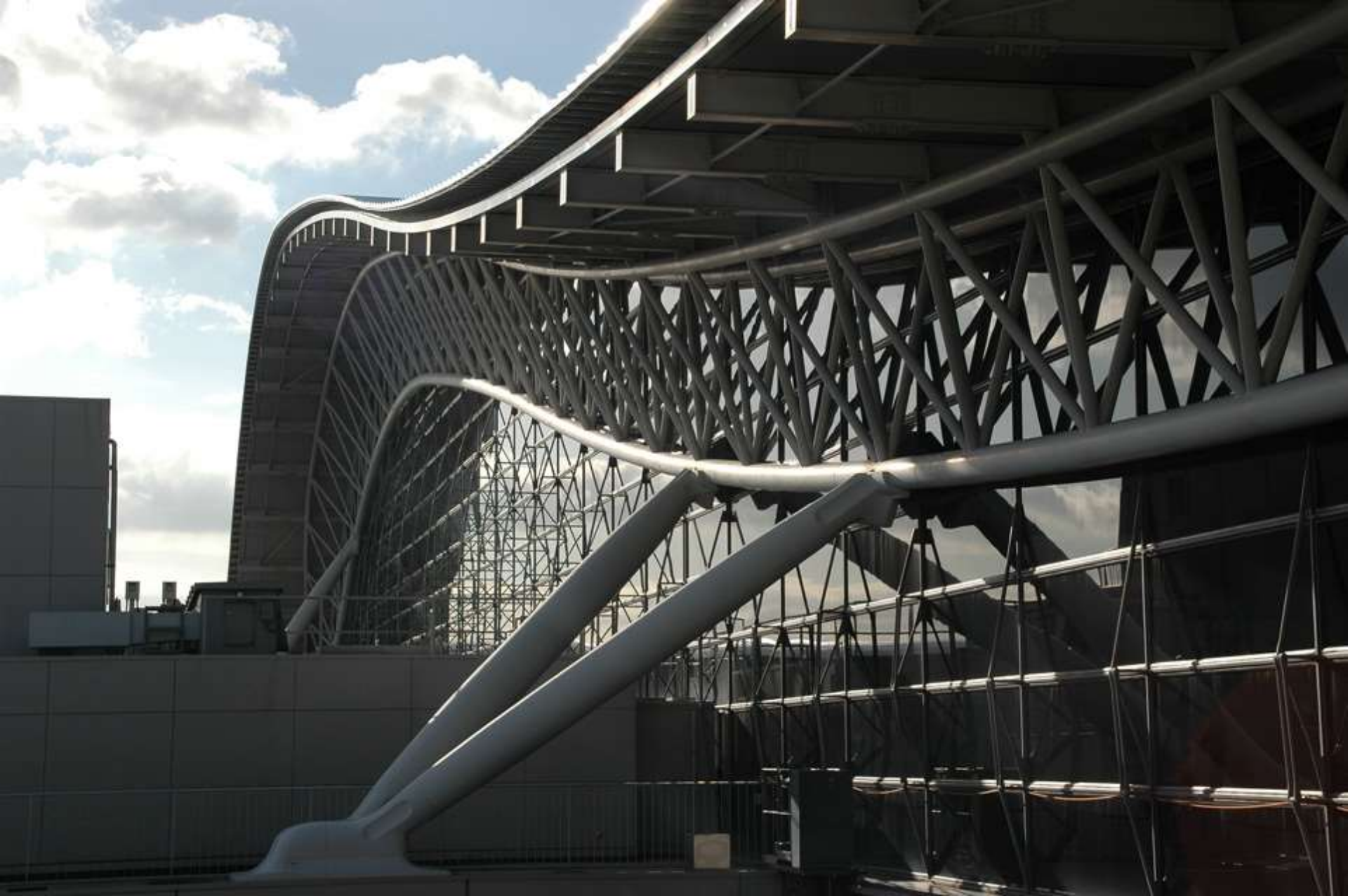
Airport Terminal, Osaka, Japan, Renzo Piano, 1994
